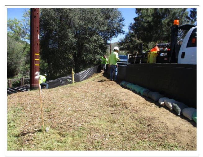
**Photo 1:** A construction crew was observed installing silt fence at Pole Z172800 (TL 629A) in accordance with the Erosion Control Plan (MM HYD-1) and was installed under the supervision of the Authorized Biologist per the recommended impact avoidance and minimization measures for the line.
