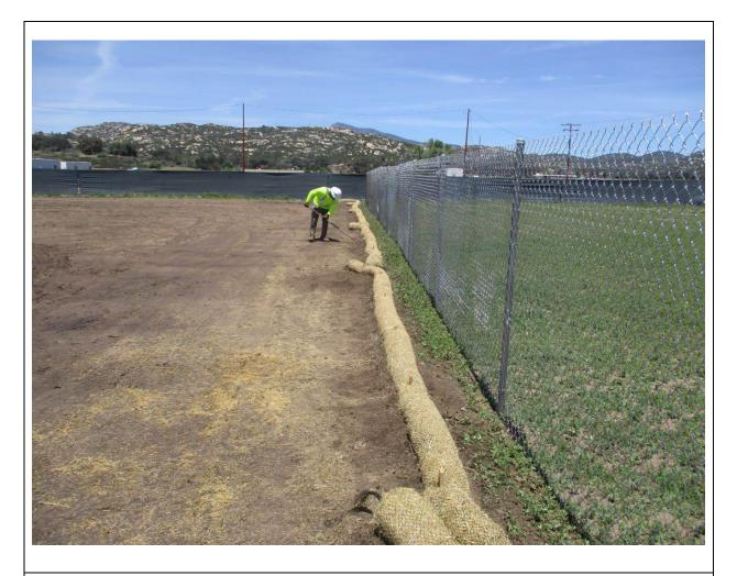
**Photo 2:** A crew member was observed finishing the installation of BMPs (straw wattles) along the perimeter of Merrigan Staging Yard expansion on TL 629A in accordance with the Erosion Control Plan and SWPPP. Opaque visual screening fencing was observed installed at the Merrigan Staging Yard (TL 629A) in accordance with APM VIS-02.
