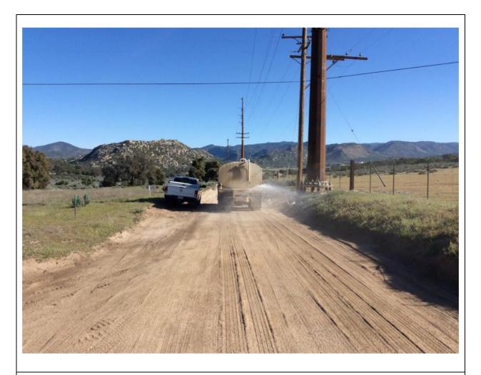
**Photo 5:** A water tender was observed applying water to the access road along TL 6958 to minimize dust emissions in accordance with APM AIR-02.
