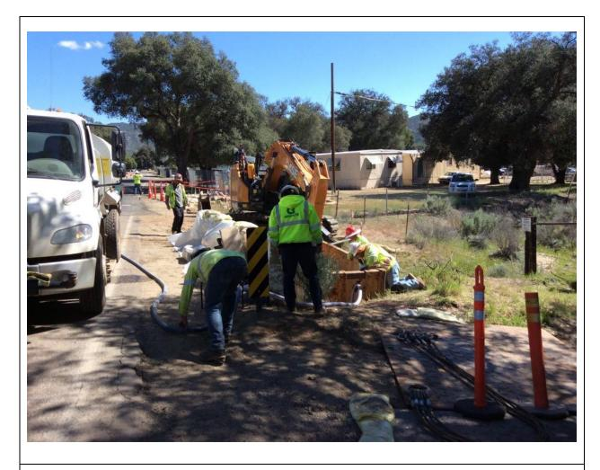
**Photo 4:** Groundwater encountered in the ephemeral stream channel near 19+96 was pumped into a water truck and later dispersed onto Morena Stokes Road on C 449 in accordance with APM HYD-08 and MM BIO-1.
