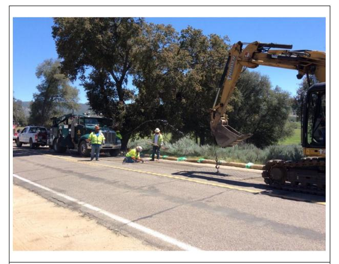
**Photo 3:** A dedicated fire patrol was observed wetting down the area surrounding hot work near along C449 and a complete set of fire tools was staged on site (5-gallon backpack pump, round point shovel, Pulaski, and 2A10BC fire extinguisher) in accordance with the CFPPP (MM FF-1).
